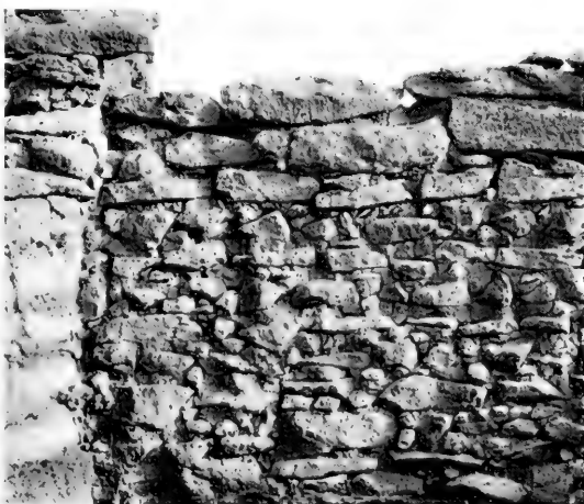
Illustration of the masonry at Pueblo Kotyiti. The larger blocks of stone were roughly dressed with stone tools and laid in mortar, after which the wall was chinked with small angular fragments, plastered and often white-washed
